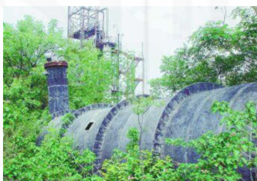
Fig.3.7: The methyl isocyanide tank at Union Carbide Corporation's factory in Bhopal, which leaked in December 1984 causing a major disaster. Waste material dumped in and around the factory is now feared to cause soil and groundwater contamination in the neighbourhood of the site. (Source: http://www.flonnet.com/ )
