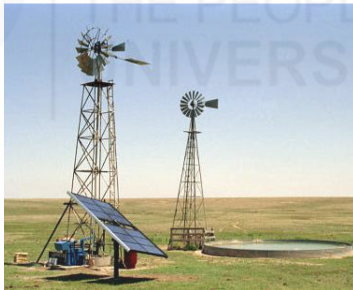
Fig.13.14: A hybrid system for water pumping
