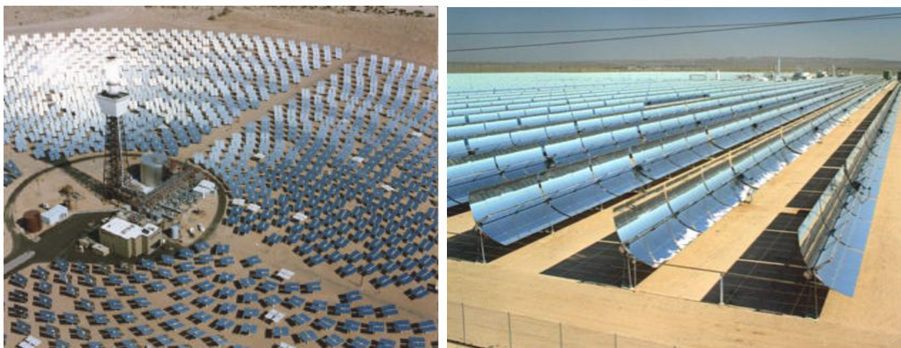
Fig.13.8: Solar thermal power plants with tower type and trough type collectors
