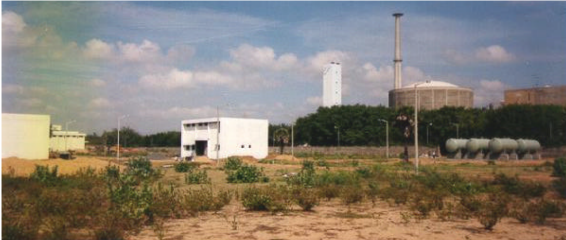
Fig.3.8: The Kalpakkam nuclear plant
