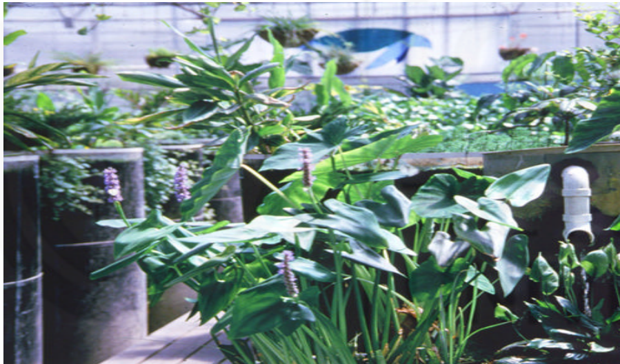
Fig.16.1: Living machines are complex ecosystems which can be used for wastewater treatment
