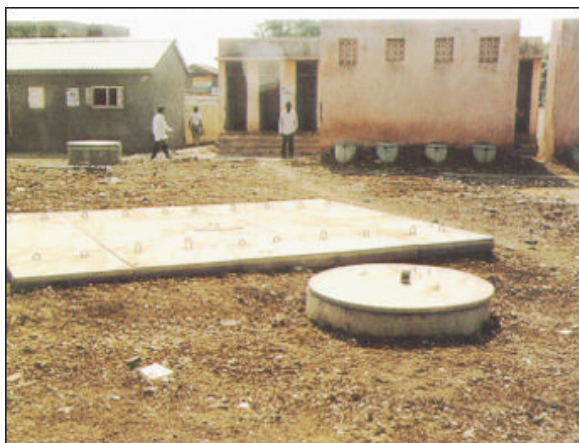
Fig.9.14: A biogas plant
